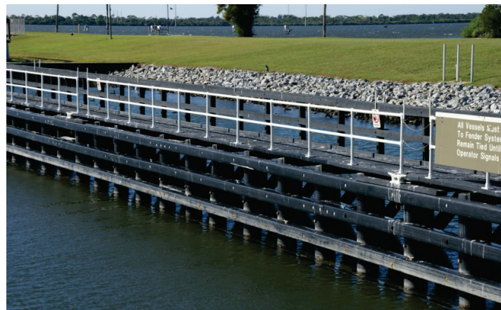
Composite timbers installed on a lock guidewall
