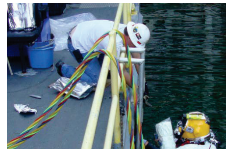
Worker handing diver a roll of composite wrap
