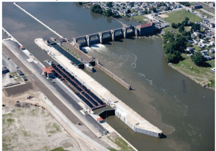
Figure 1: A new 110' x 800' lock chamber, completed in 2009 at Marmet Locks and Dam, adds vessel handling capacity to the two original 56' x 360' chambers, constructed circa 1933, to help alleviate traffic delays on the Kanawha River.
