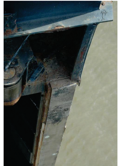
Miter block with epoxy backing material
