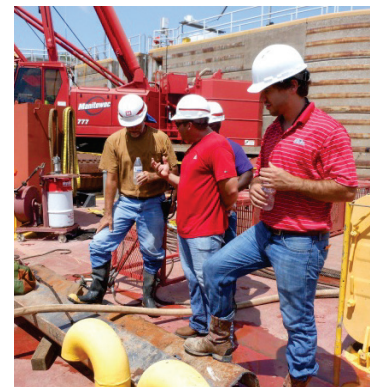
Concrete repair operations at Newt Graham Lock and Dam
