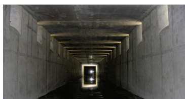
Inside Marmet Lock culvert
