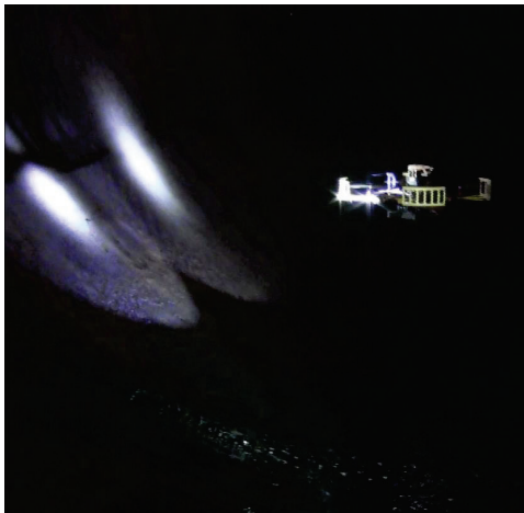
Quadrotor operates in penstock at Carter's Dam, Georgia
