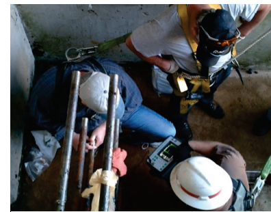
Tension testing of rods at West Point Dam, GA
