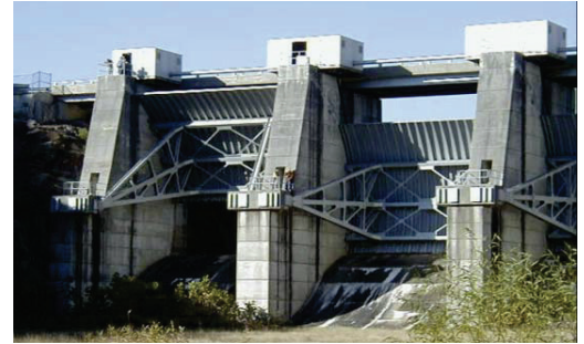
West Point Dam, GA
