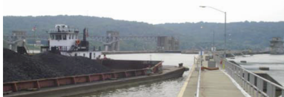
Barge train impacting a flexible approach wall
