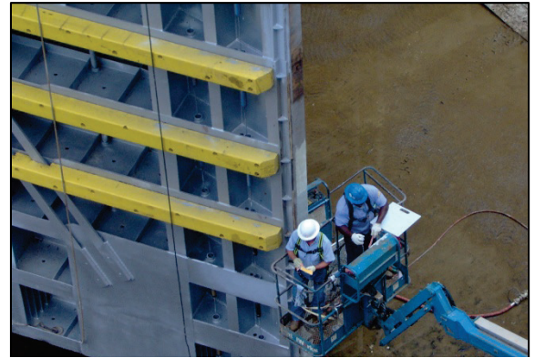
Plastic timbers being mounted on a miter gate
