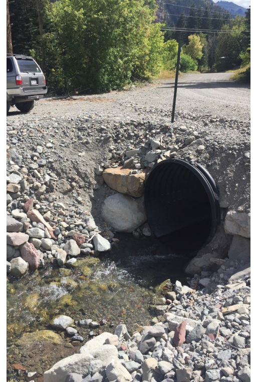
Existing culvert under CR-17. (Kellie Jemes, 2019)
