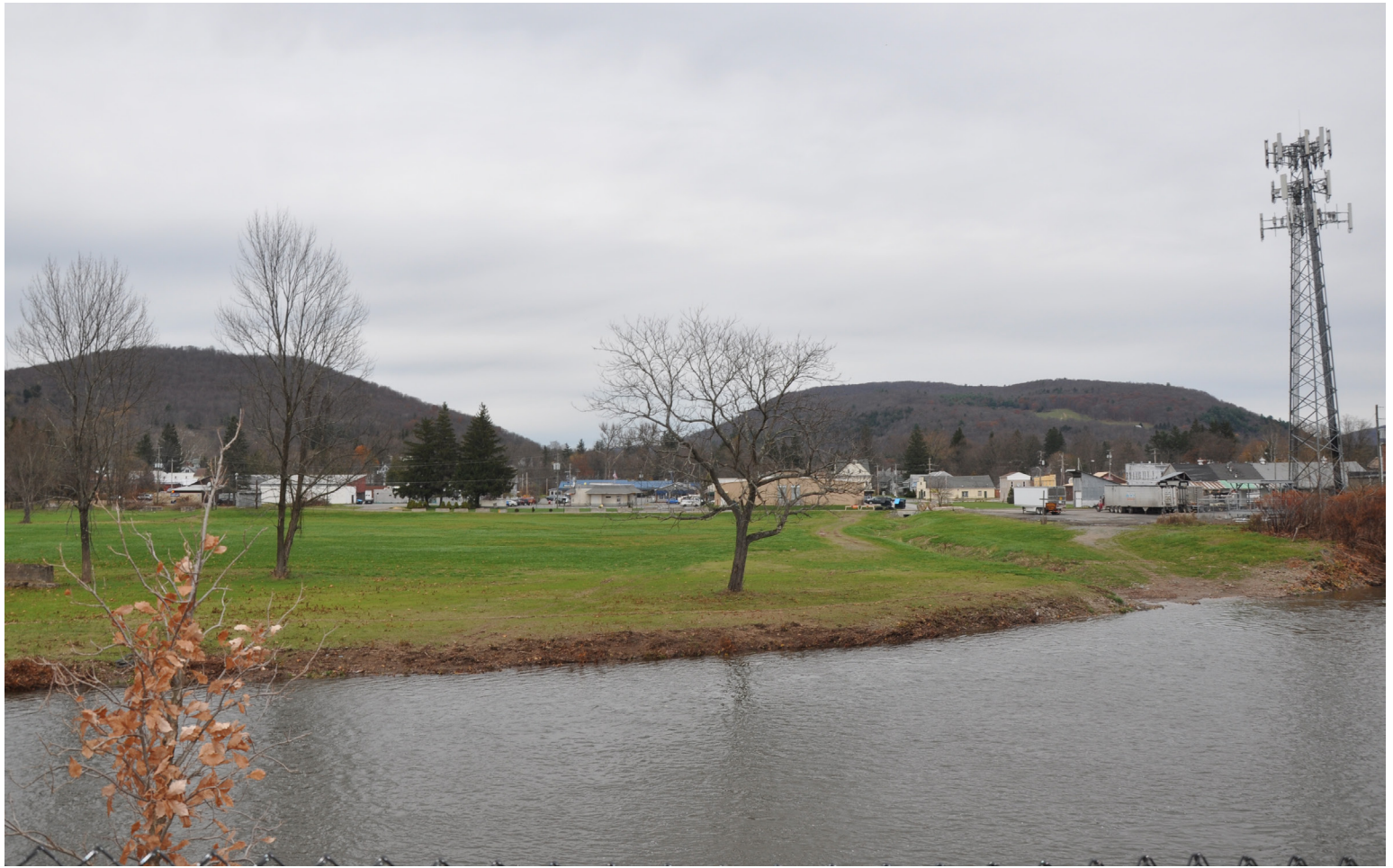
“After” photo: The completed Walton floodplain project. (JoAnne Castagna, 2019)
