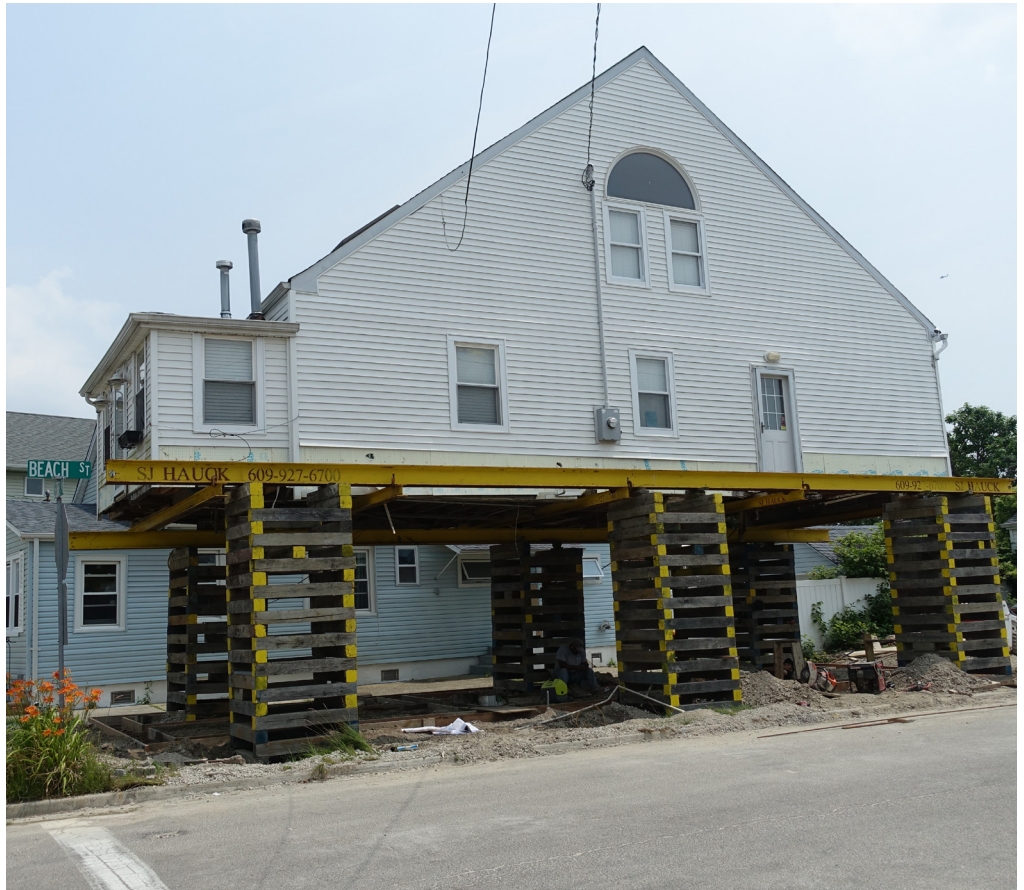
An example of elevation, a nonstructural technique, as part of Hurricane Sandy recovery in New York state.
