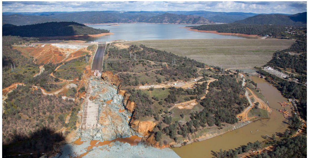
Oroville Dam spillway erosion, 2017.
