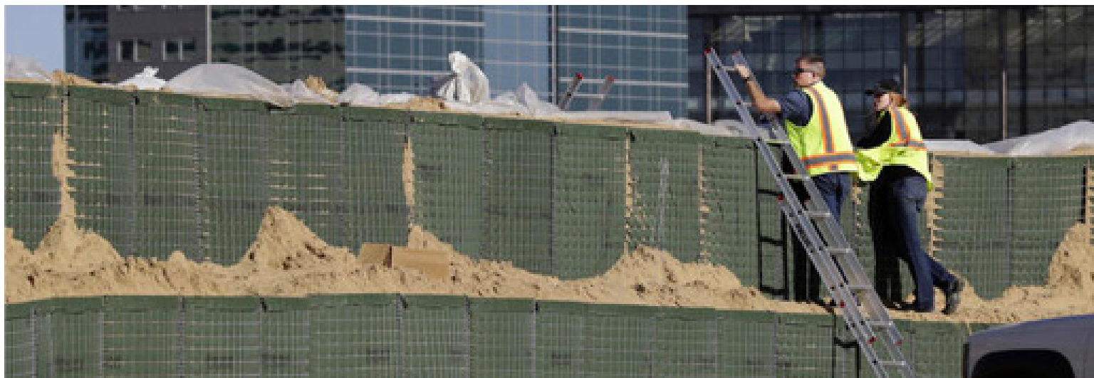
Workers stand on a flood wall made of Hesco barriers on the bank of the Cedar River, Monday, Sept. 26, 2016, in Cedar Rapids, Iowa. (Charlie Neibergall / AP).
