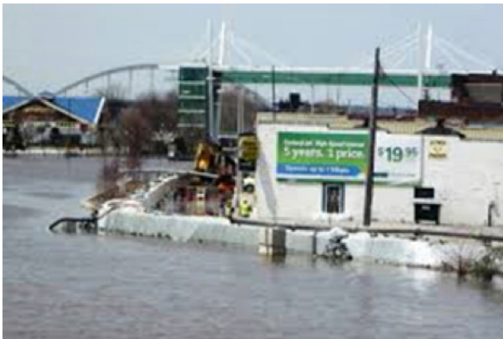
Temporary setback levee constructed of Hesco Barriers along Front Street in Davenport, Iowa.
