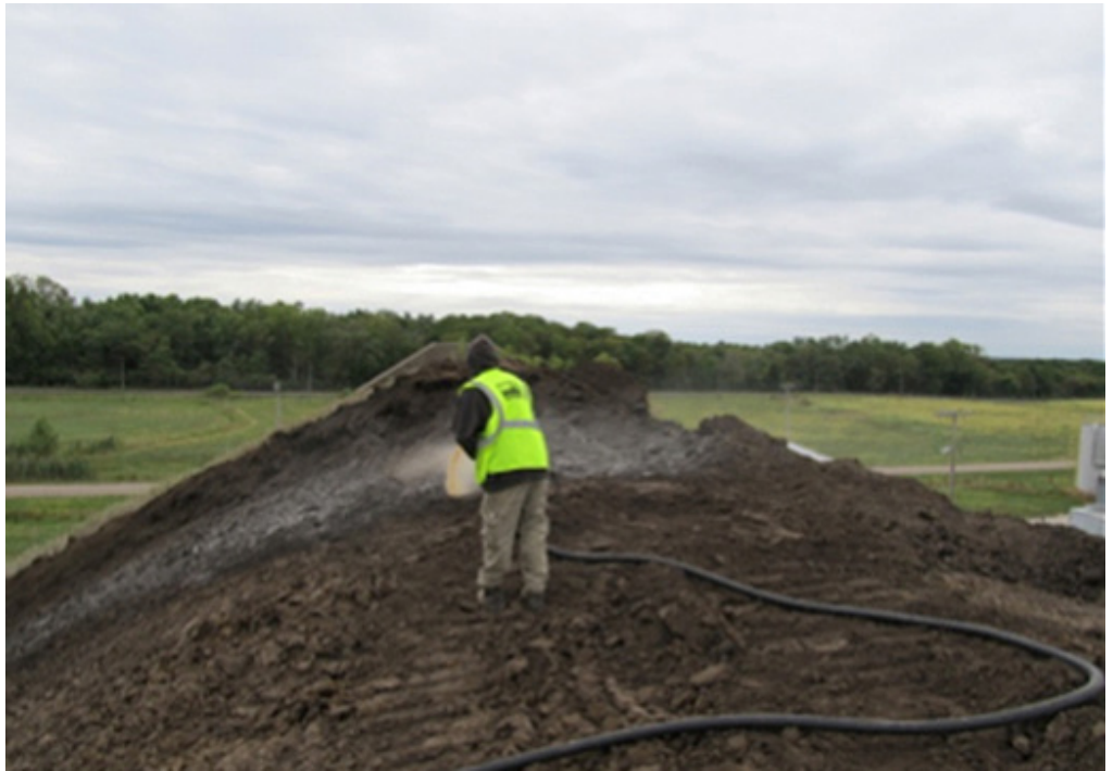
Liquid EPS biopolymer being applied to a test levee with grass seed using standard hydroseeding equipment.
