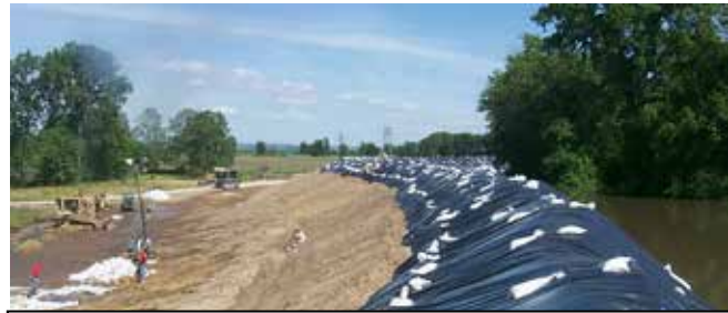
Completed sand levee “push-up” during record 2008 flooding
