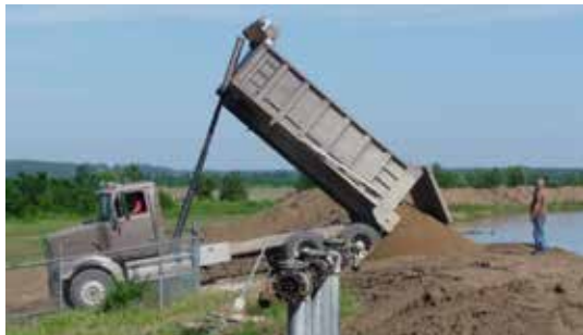
Dumping additional sand on mainstem levee during record 2008 flooding
