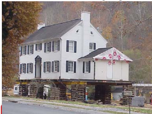
Elevation – raising in place
