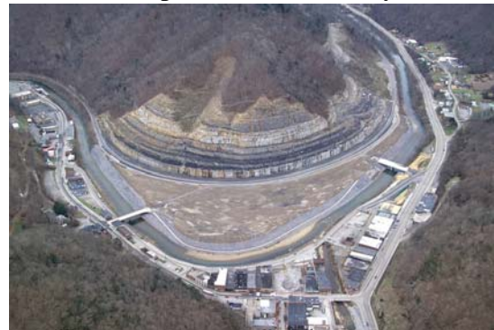
Redevelopment site – Grundy, VA
